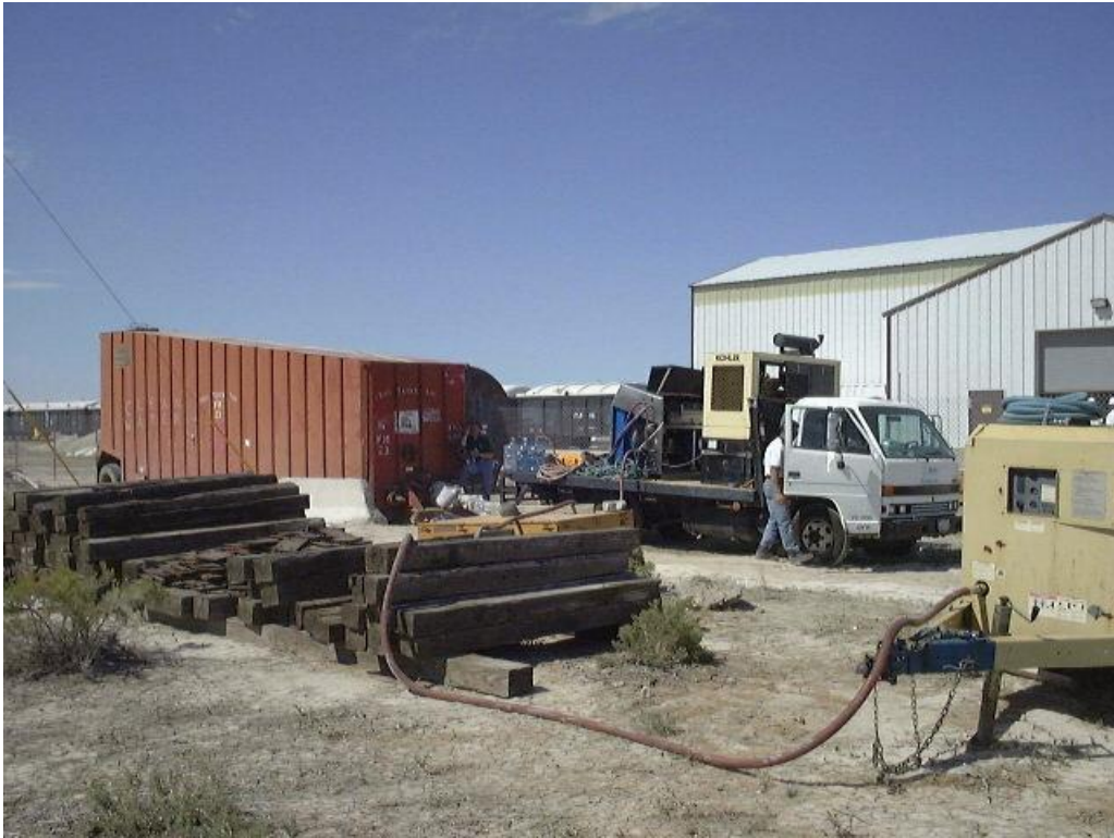
Picture 4: Mobile ice blast system inside buffer zone.
